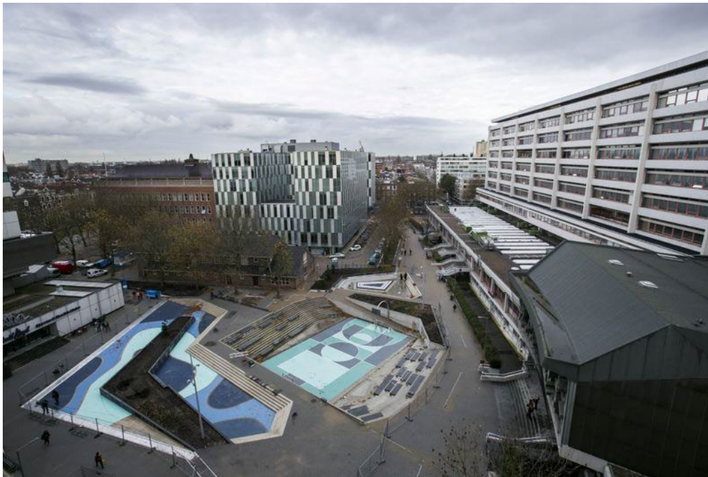
Figure 24: Rotterdam's Bentheplein water square is used as an amphitheater, basketball court, or skateboarding rink in good weather. When a cloud burst hits it transforms into a series of collection ponds.
