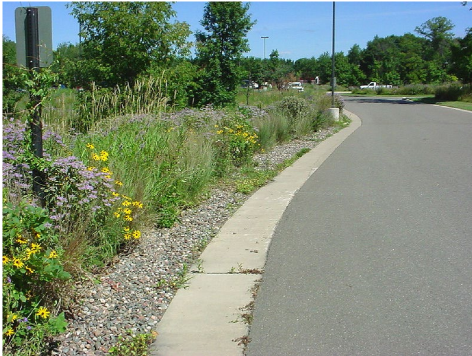
Figure 21: A raised curb has been removed and sheet runoff runs directly into an infiltration trench and bioswale.
