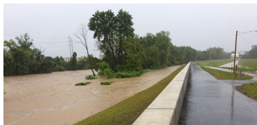
Figure 26: This floodwall is successfully keeping floodwaters away from a pedestrian path.
